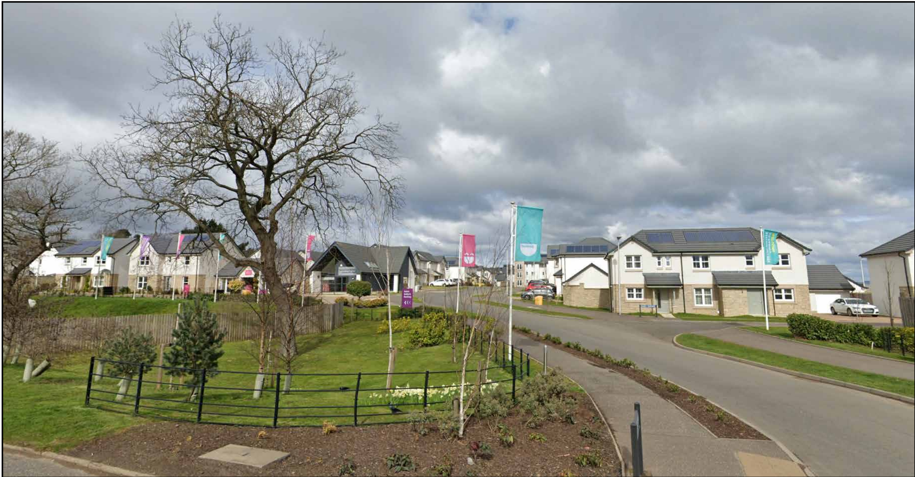
Dundas Estates development at Uphall Station Village
